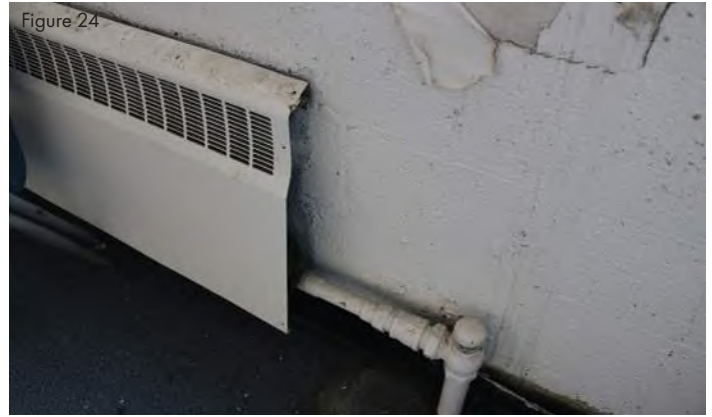
Classroom radiator cabinet missing end caps.
