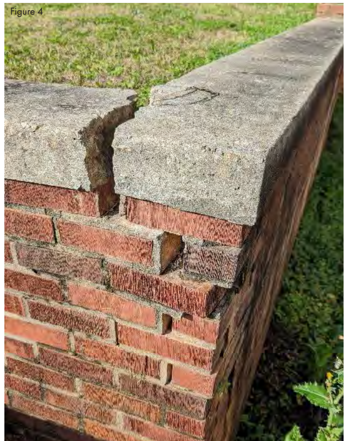
Masonry retaining wall failing
