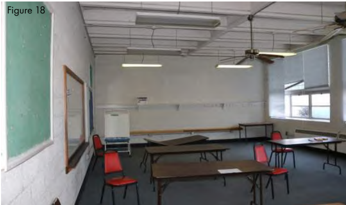
Typical Original Building Classroom Lighting. Several fixtures are not operating.
