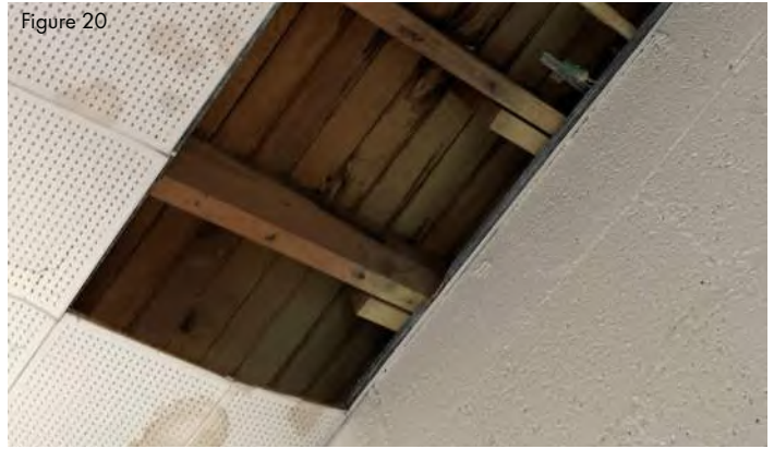
Damaged and missing ACT in gym
