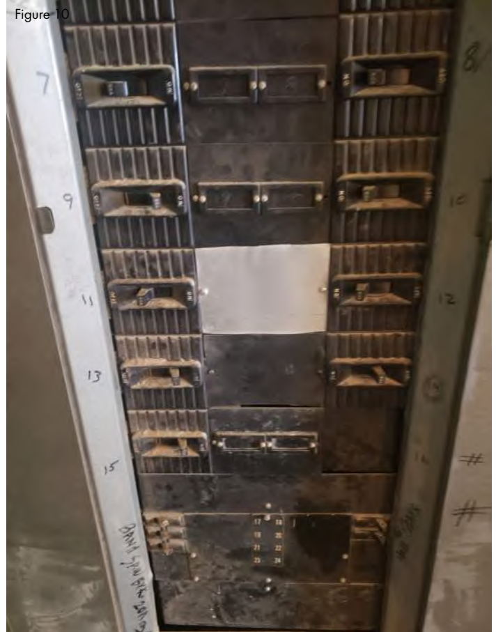
General condition of the interior of the gymnasium panels is dirty and dusty.
