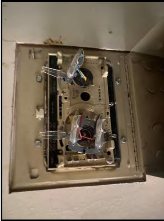
13 Mercury thermostat in the cafeteria.
