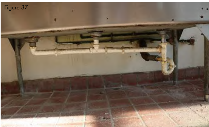
Kitchen three compartment sink waste piping.
