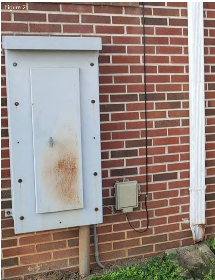
South wing exterior surface mounted panel is rusting.
