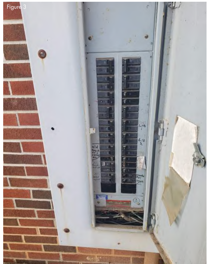
Interior south wing of electrical panel missing escutcheon and has dirt, cobwebs and debris inside.
