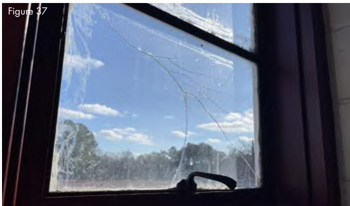
Damaged glazing should be replaced
