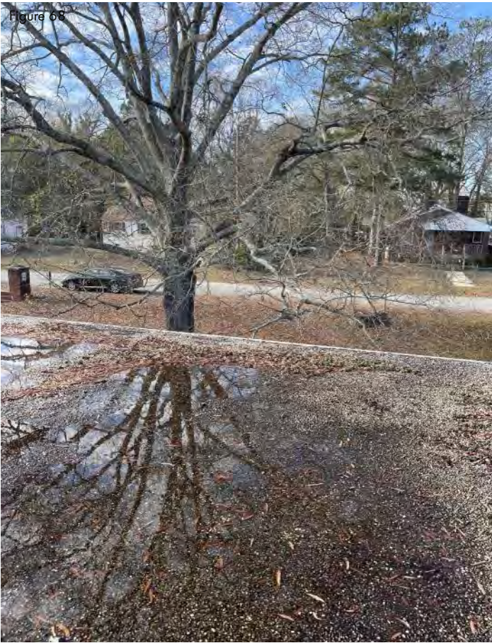
Ponding on roof
