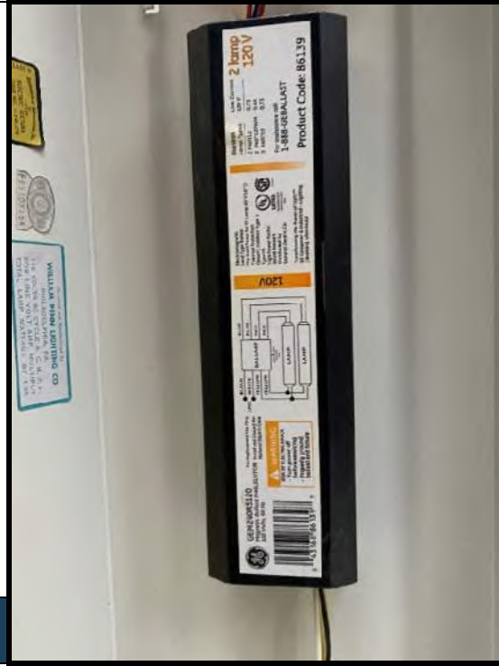
16 Electromagnetic ballast no PCBs.
