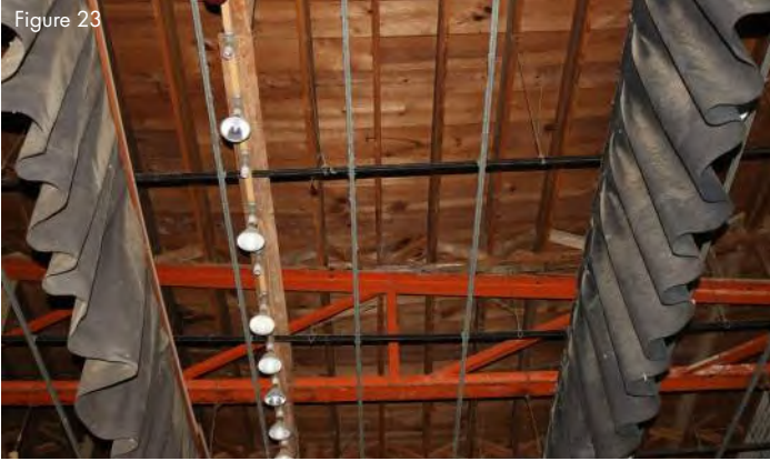
Stage Lighting. Several sockets do not have bulbs installed.
