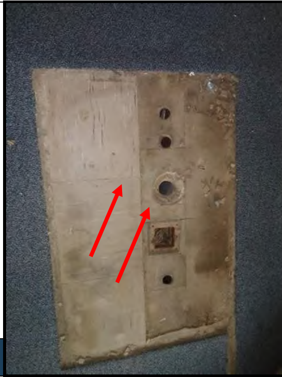
3 12-inch dark tan vinyl floor tile and black mastic and 9-inch brown vinyl floor tile and mastic tested positive for asbestos (3%-6% chrysotile).
