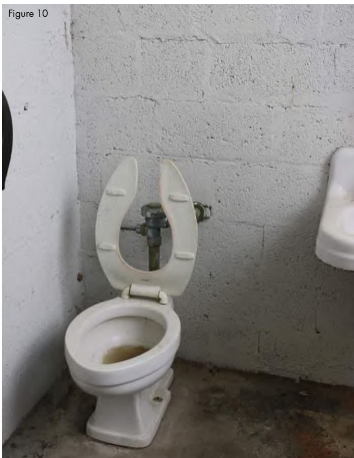
Typical flush valve toilet.
