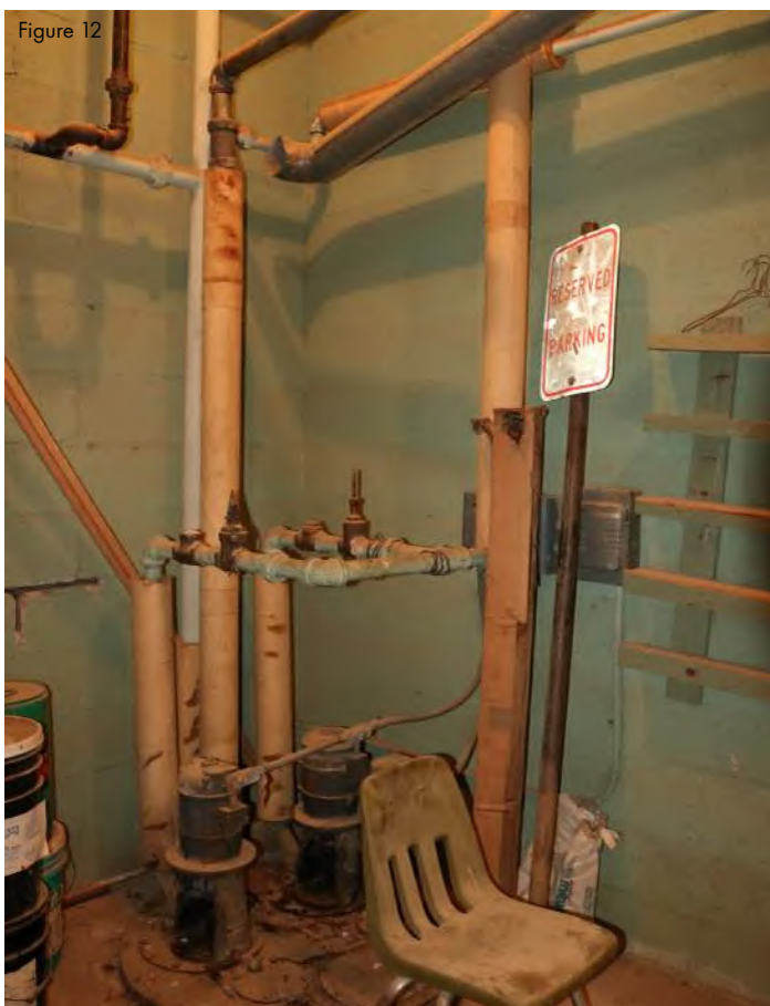
Steam condensate return pumps in fair condition. Could not verify age or operation but equipment has exceeded its normal service life.
