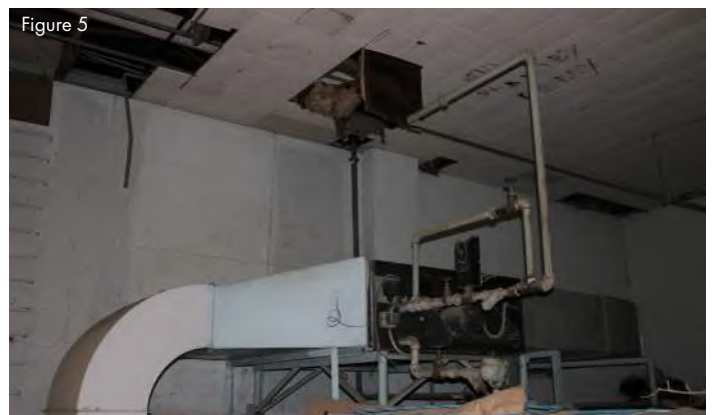
Figure 5 Gym heating unit #2. No cooling. Could not verify age or operation but equipment has exceeded its normal service life.
