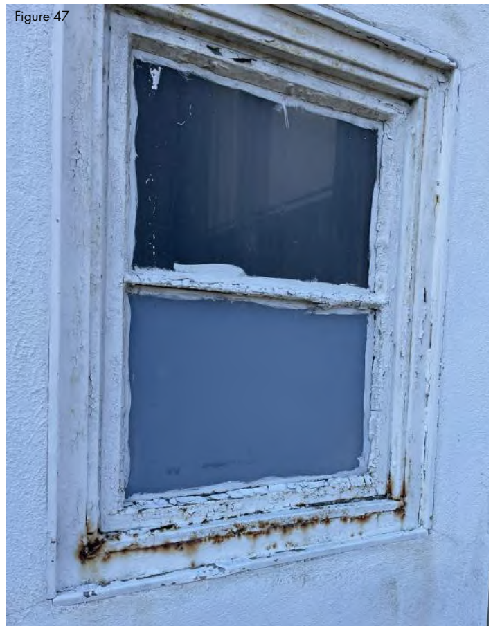
Steel window condition
