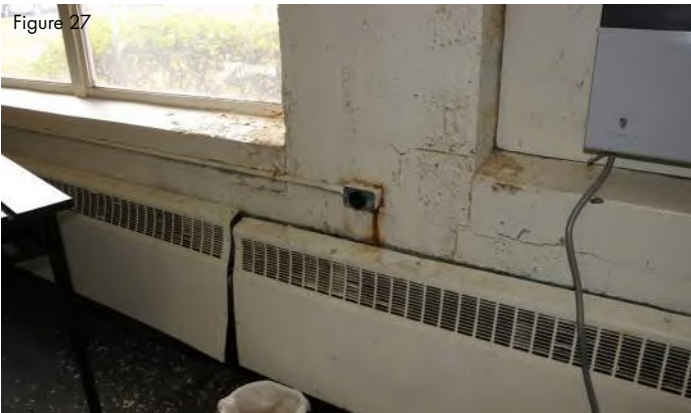
Classroom radiator cabinet damage.
