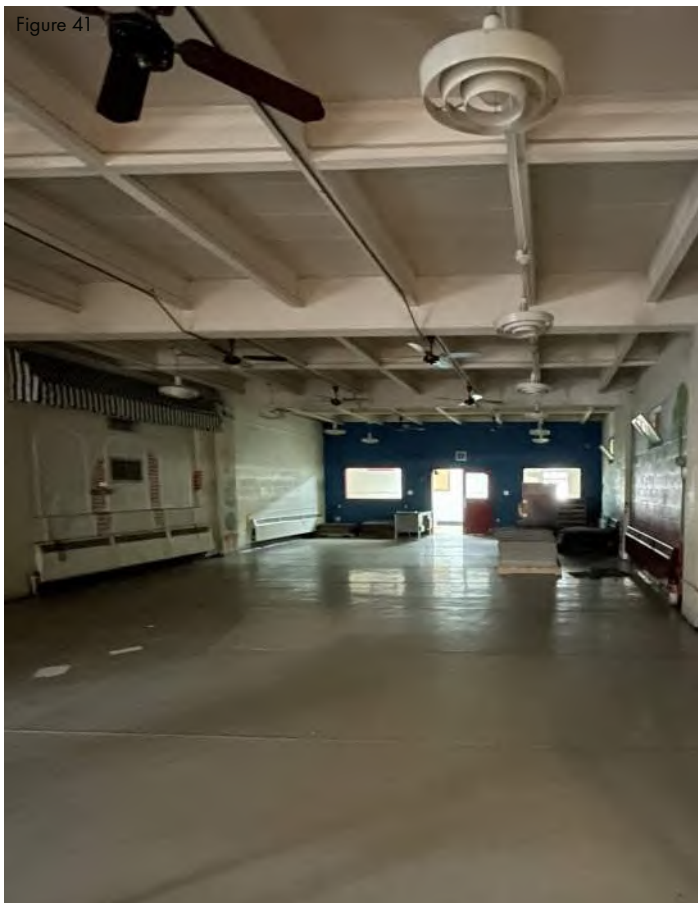
Exposed ceiling in cafeteria - underside of concrete roof deck & concrete joists
