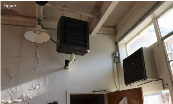
Figure 1 Kitchen heated with fan forced heater suspended from the roof structure.
