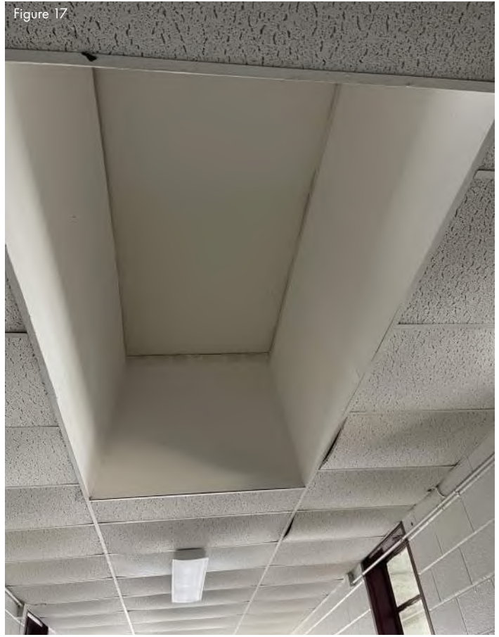
Original opening for skylight - Wasco Skydome (original drawings)
