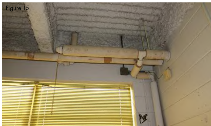
Gaps in the piping insulation need to be addressed.
