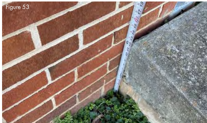
Ramp with approximate 12" rise - anything greater than 6" should have railing
