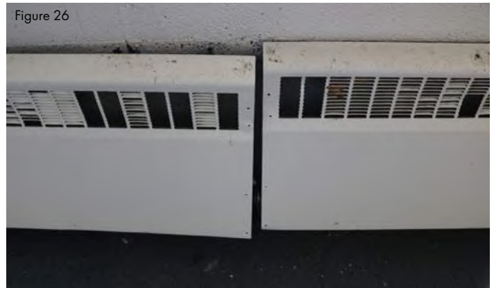
Classroom radiator cabinet damage.
