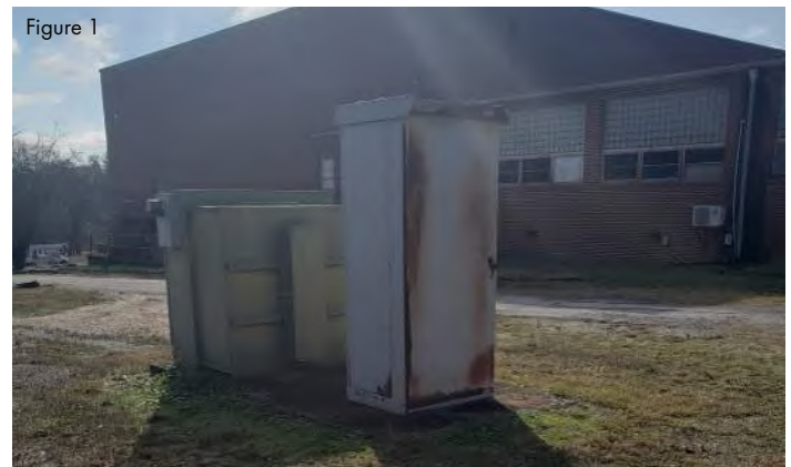
Transformer and Distribution panel are rusting and showing signs of age.
