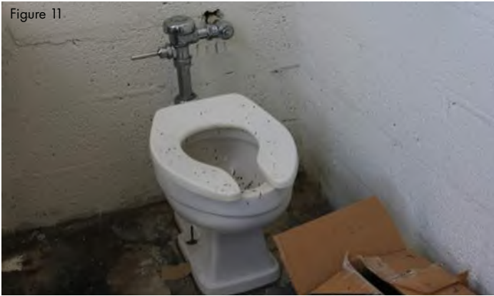
Typical flush valve toilet.
