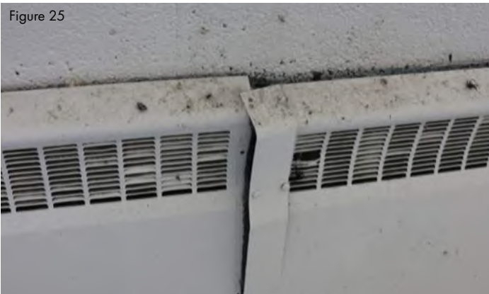
Classroom radiator cabinet damage.
