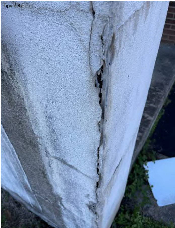
Rusting metal components and spalled stucco
