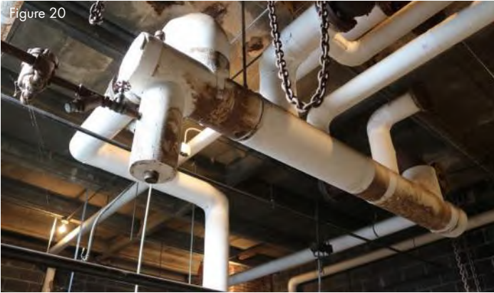
Roof leaks damaging pipe insulation. Insulation needs to be replaced.
