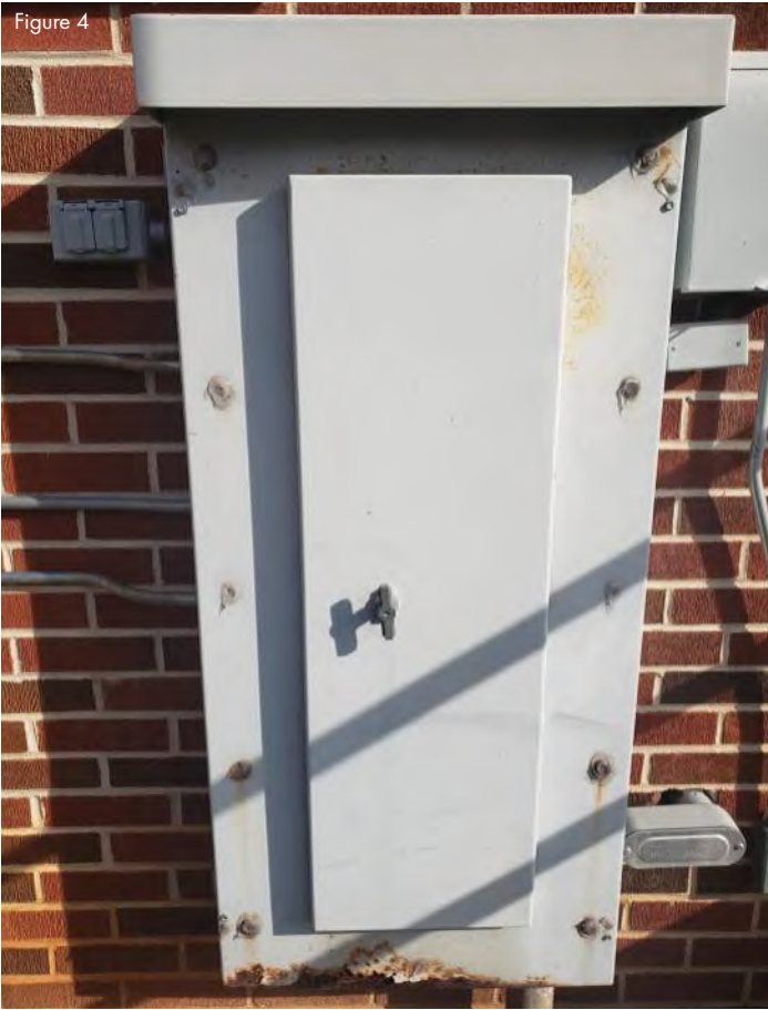
North wing exterior surface mounted panel is rusting.
