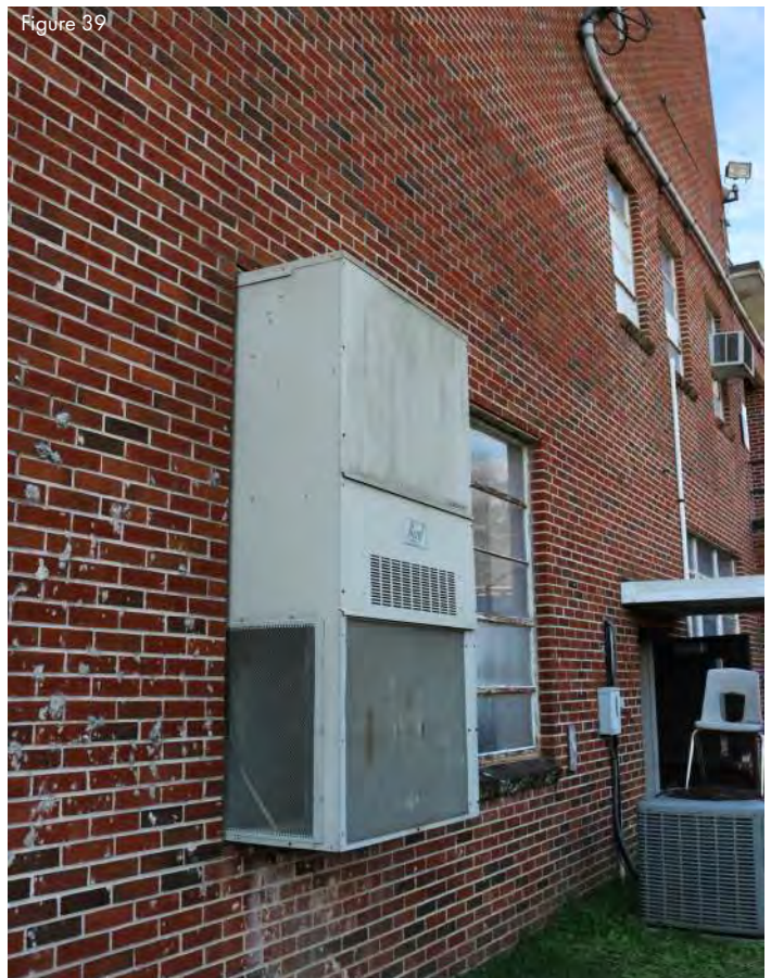
Exterior view of Lower-level Office area Bard air conditioning unit.
