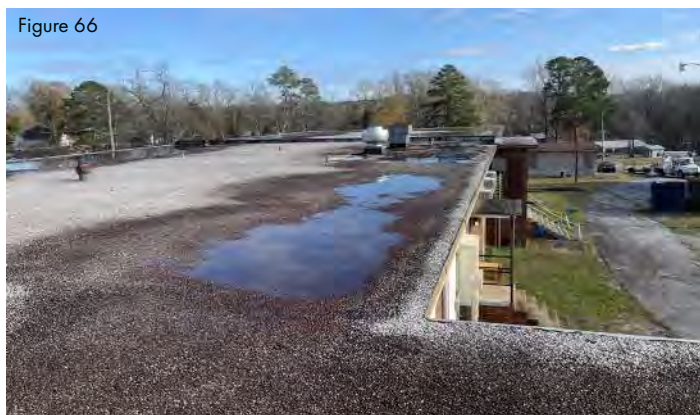
Ponding on roof
