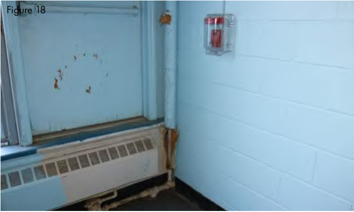
Lower-level classroom stairwell needs to have pipe insulation replaced.
