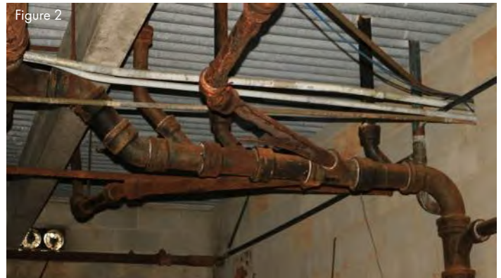
Cast iron pipe under expansion gang toilets needs to be replaced.
