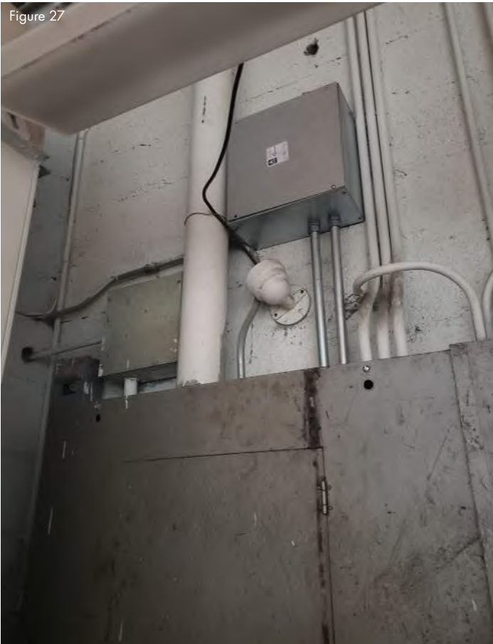
Light fixture was reworked in an unconventional manner to provide power to a light strip.
