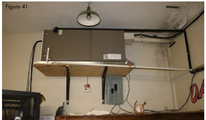
I.T. room split system air handler in good condition. Note moisture issue on right hand wall.
