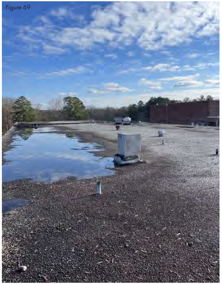
Ponding on roof
