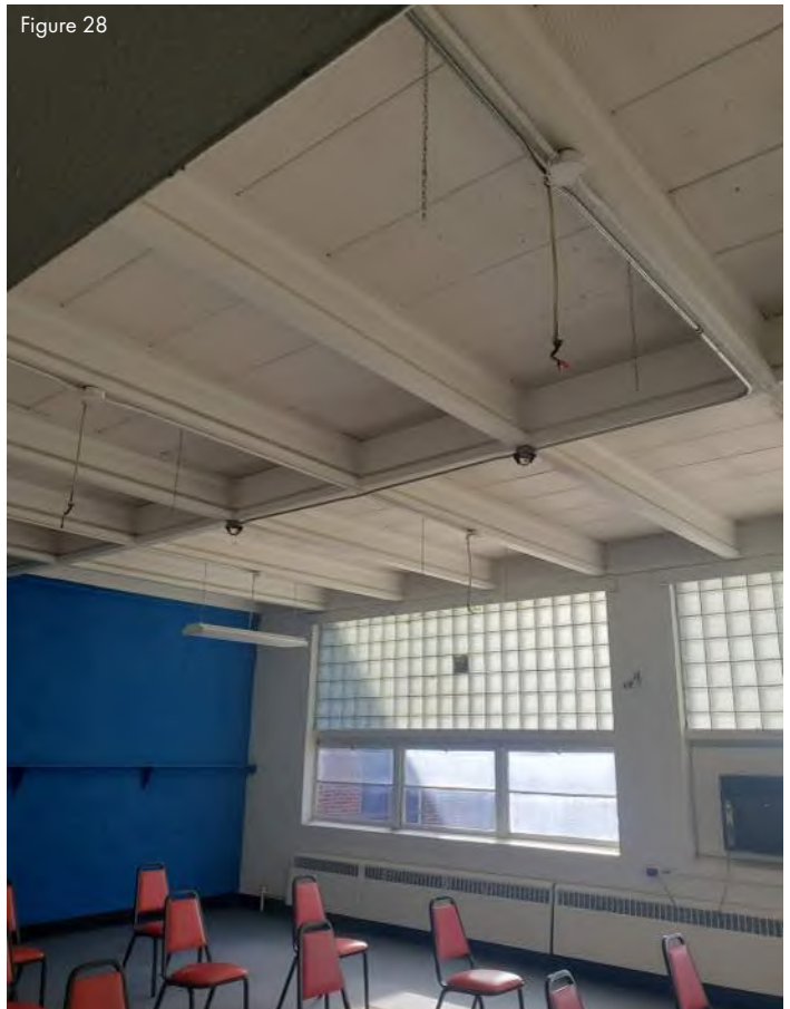
Typical lighting and ceiling fan circuitry not terminated properly.
