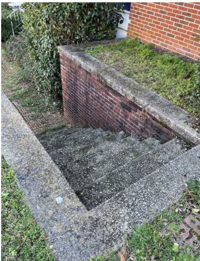
Exterior stair on site adjacent to gym - notice no handrail
