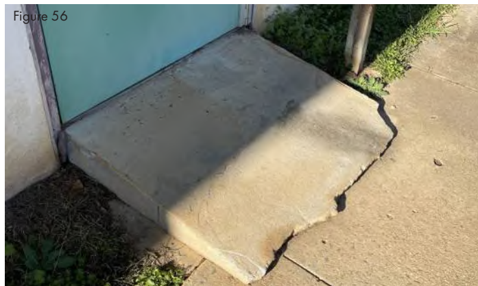
Not an accessible path into the ground floor of the addition
