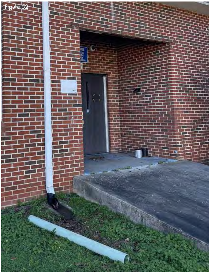
Ramp with approximate 12" rise - anything greater than 6" should have railing
