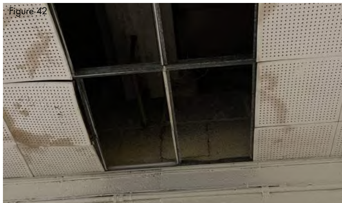
No insulation above the acoustical ceiling tiles in corridors
