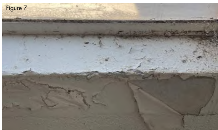
Evidence of moisture infiltration at exterior walls
