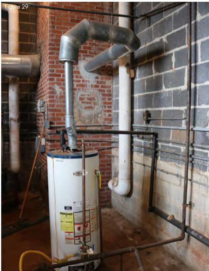
Figure 29 Chimney should be inspected if it is to be reused in the future for boiler and water heater flues.
