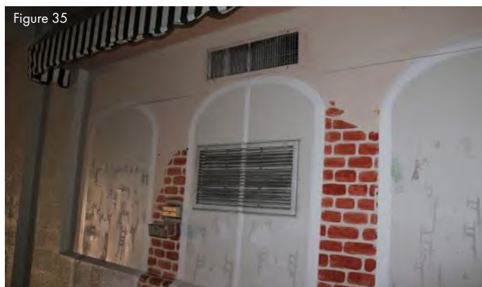
Figure 35 Cafeteria Bard unit supply and return grilles need to be cleaned and are in good condition.
