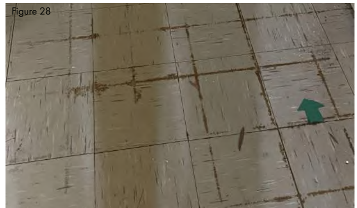
Figure 28 12x12 VCT over 9x9 asbestos tile in corridor
