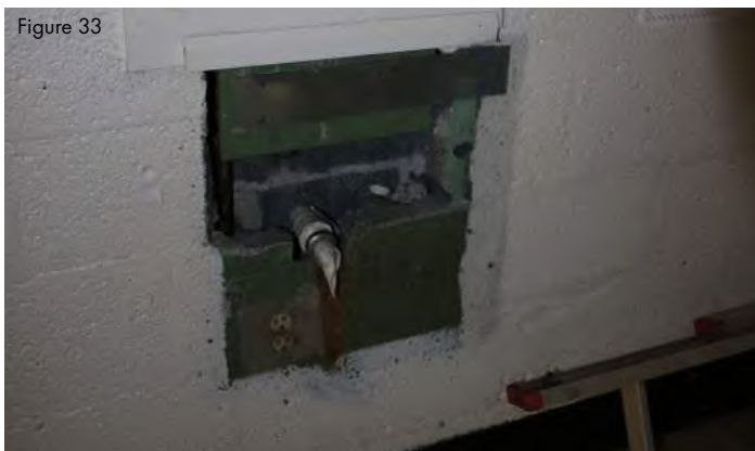
Abandoned corridor water cooler piping.
