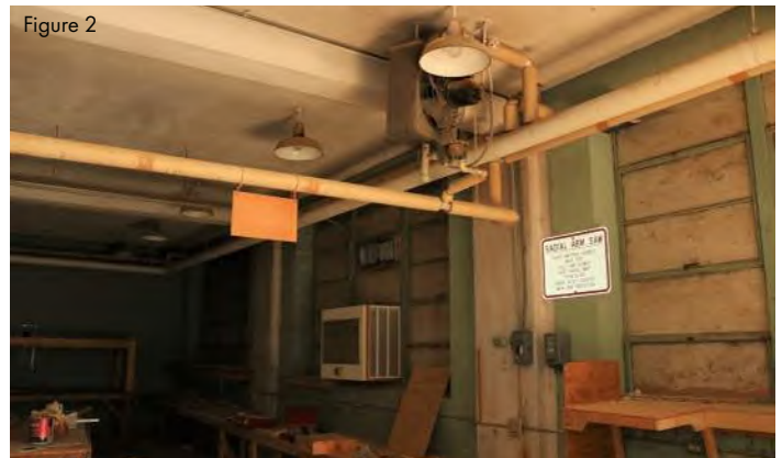
Figure 2 Shop area heated with two fan forced steam unit heater. Heaters in fair condition. Air handler serving classroom in fair condition.
