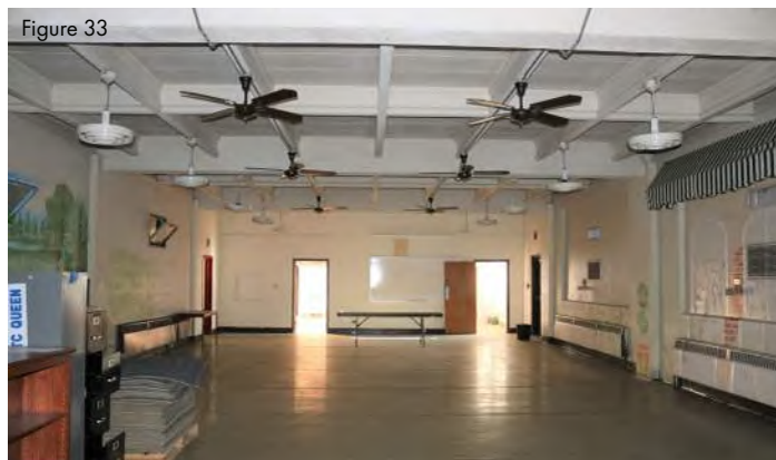
Figure 33 Cafeteria conditioned with two Bard through the wall heat pumps and ceiling fans.
