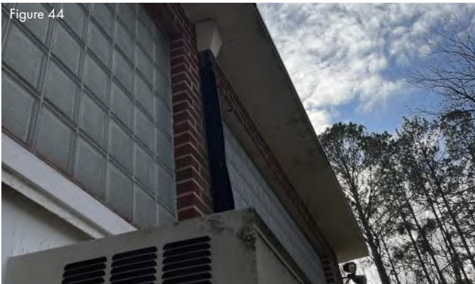
Concrete roof deck overhang
