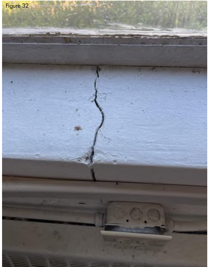
Damaged window sill
