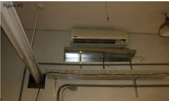
I.T. room mini-split wall mounted air handler.
