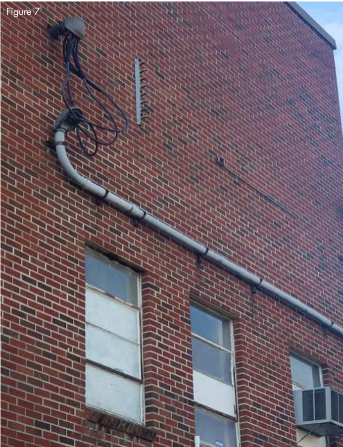
Electrical service serving the south wing is installed in an unconventional manner.
