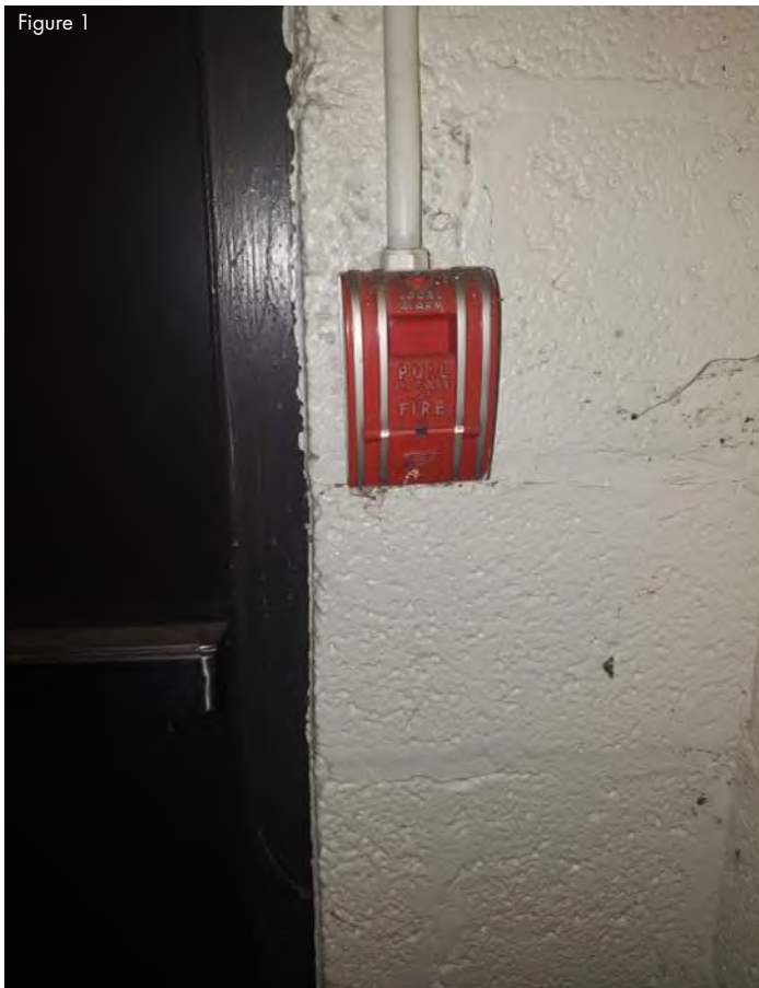
Fire Alarm Pull Station
