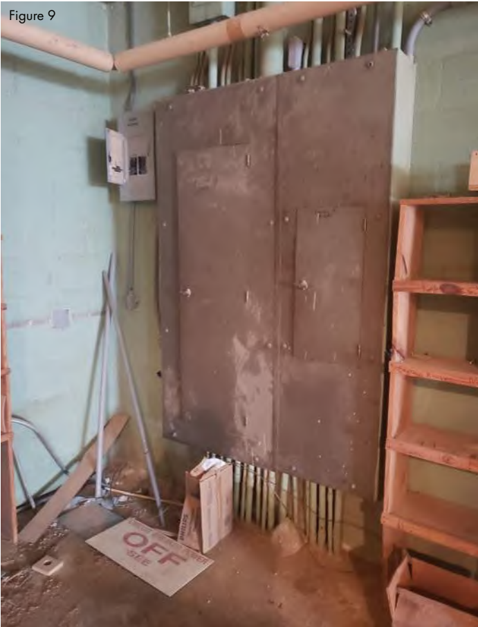
Gymnasium main and sub panel are at the end of their useful service life.
