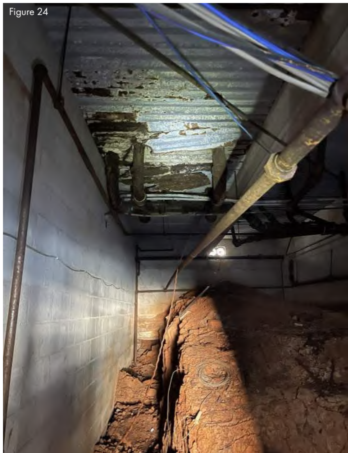
Damaged floor system from below
