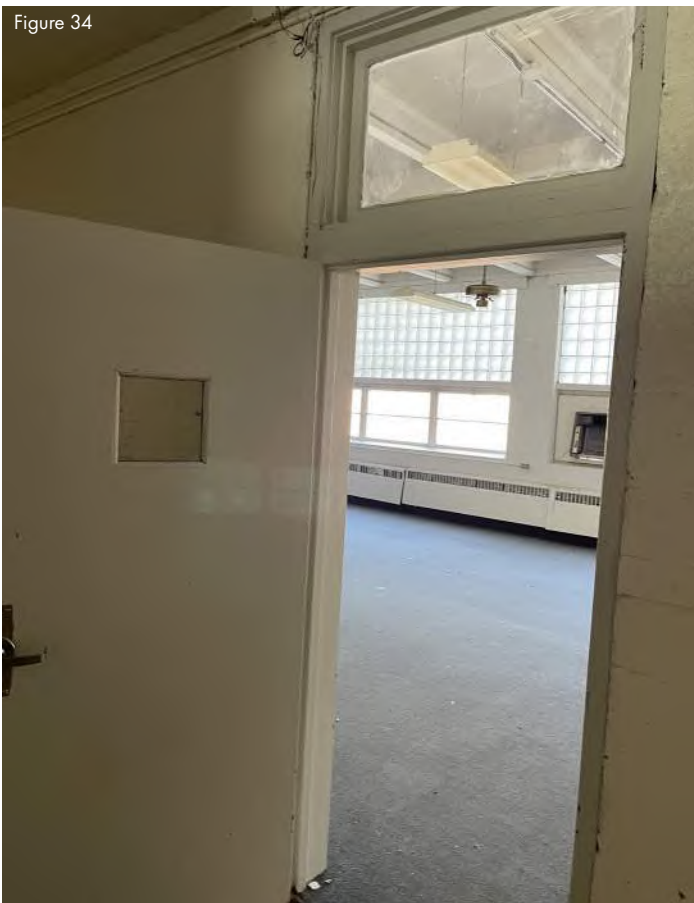
Notice the small vision glass opening and the transom
