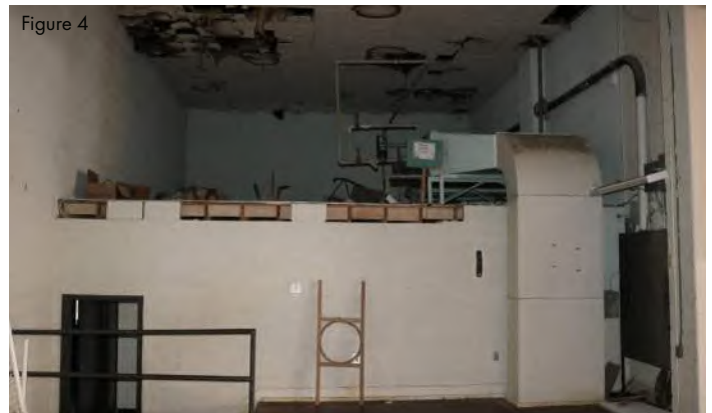
Figure 4 Gym heating unit #1. No cooling. Could not verify age or operation but equipment has exceeded its normal service life.
