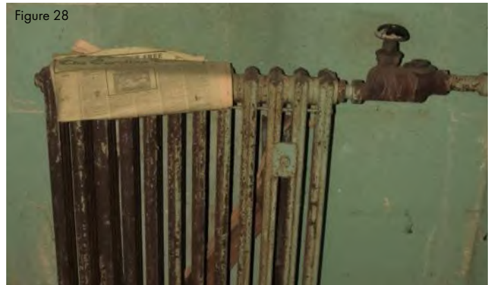
Exposed radiator in toilet/shower room. No pipe insulation. Typical.
