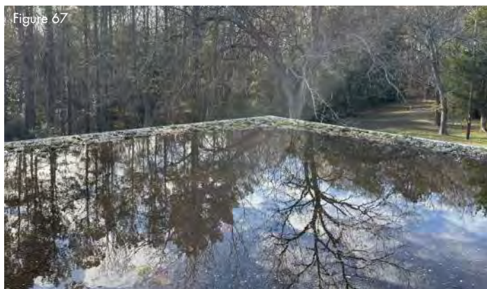
Ponding on roof
