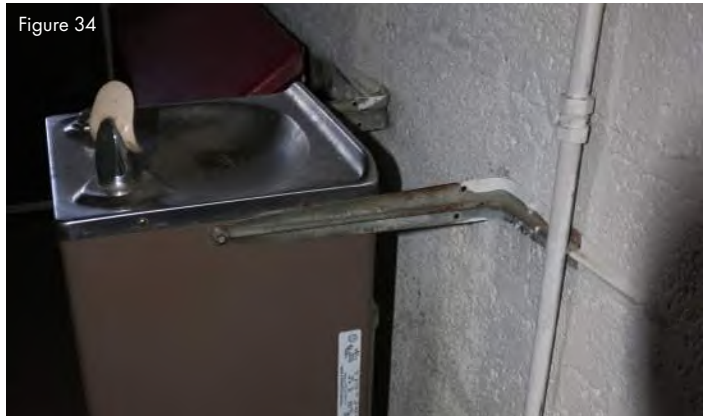
Water cooler at Gym not properly installed.
