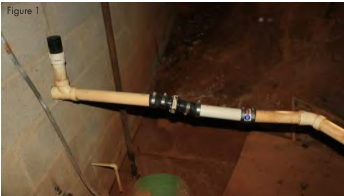
Waste piping from lower-level classroom sink needs to be replaced.
