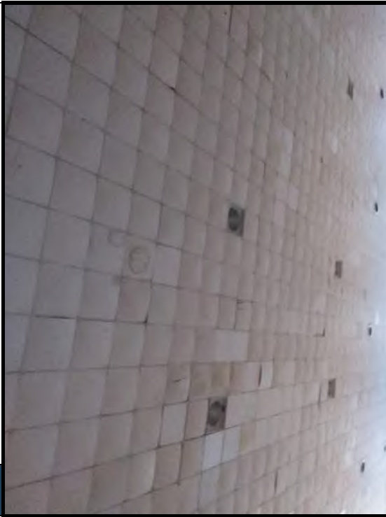
7 2x2 ceiling tile tested negative for asbestos via PLM analysis.
