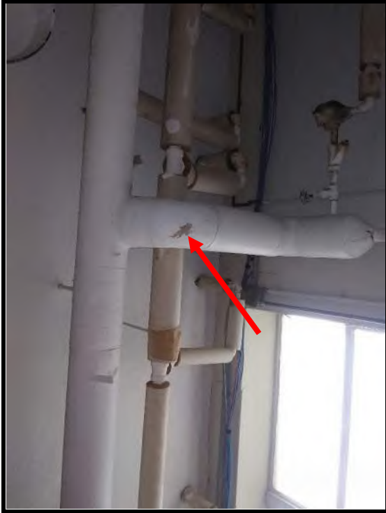
6 Hard joint tested positive for asbestos (65% chrysotile).
