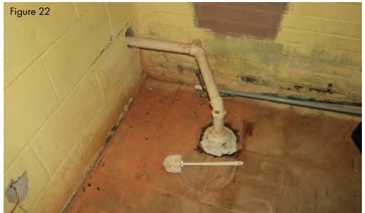
Lower level classroom wing bathroom – sink waste piped to removed toilet flange.
