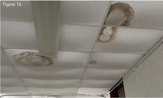
ACP ceiling - notice moisture damage
