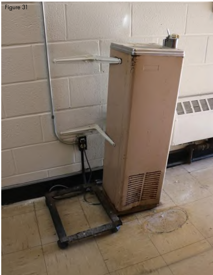
Water cooler not installed properly.
