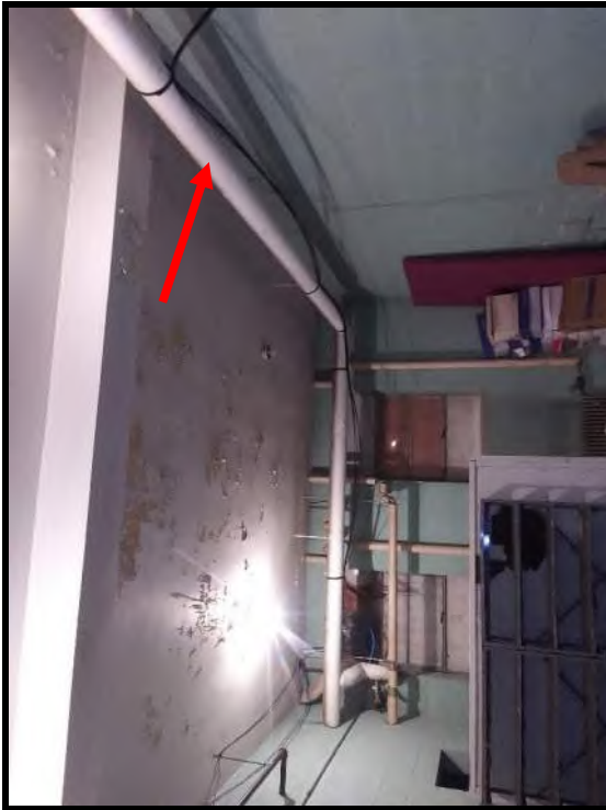
5 TSI tested positive for asbestos (15% amosite and 3% chrysotile).
