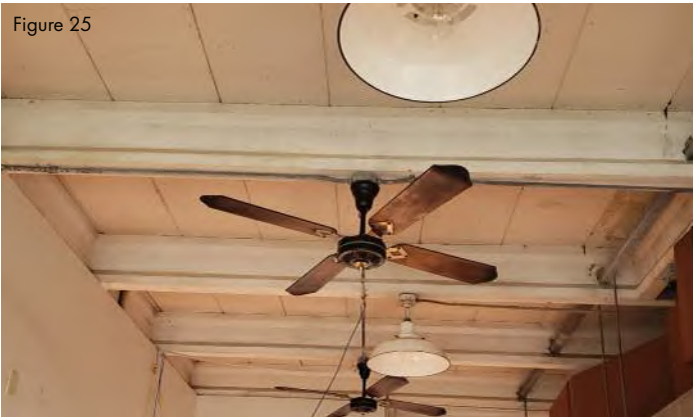
Light fixtures in the kitchen are not cleanable and don't meet current SCDHEC standards.
