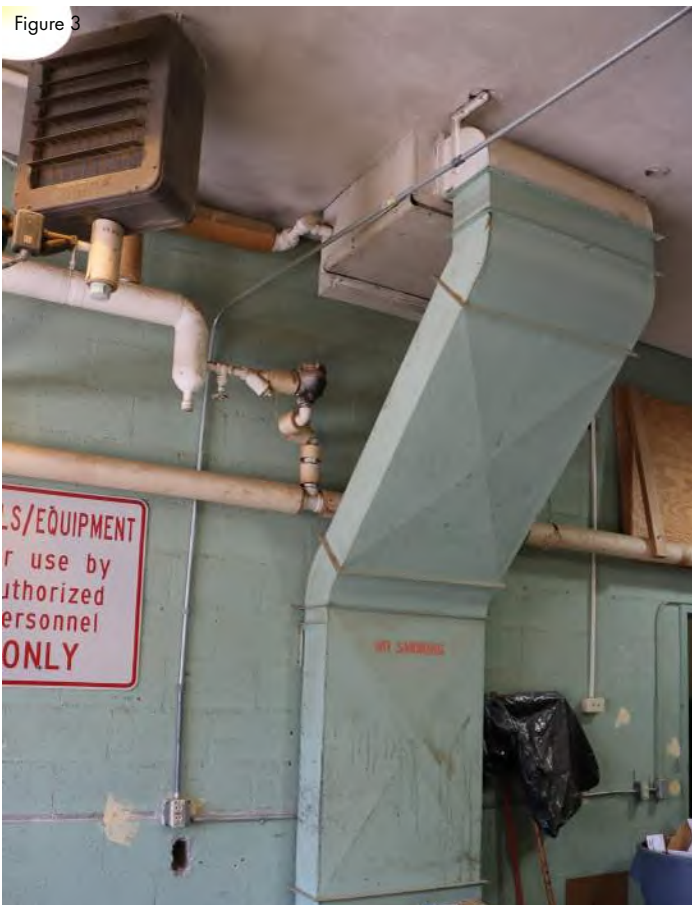
Figure 3 Shop steam unit heater #2.
