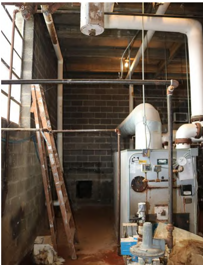
Boiler in Fair condition. Could not verify age or operation but equipment has exceeded its normal service life.
