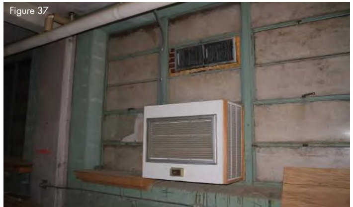
Shop Bard unit supply and return grilles. Supply grille needs to be cleaned.
