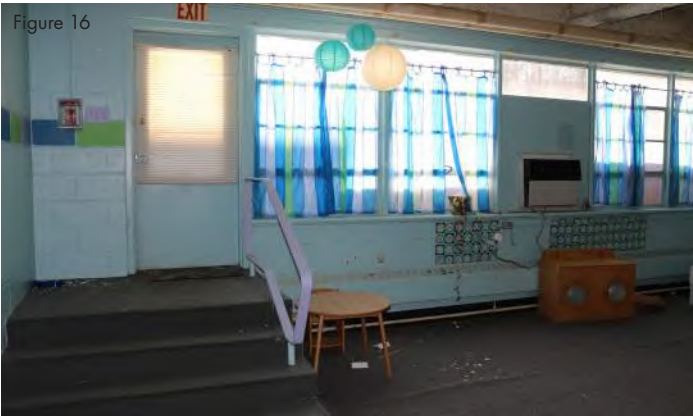
Exposed steam piping in lower-level classrooms. Window unit for cooling.
