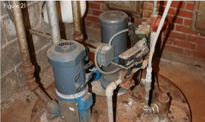
Steam condensate return pumps in fair condition. Could not verify age or operation but equipment has exceeded its normal service life.
