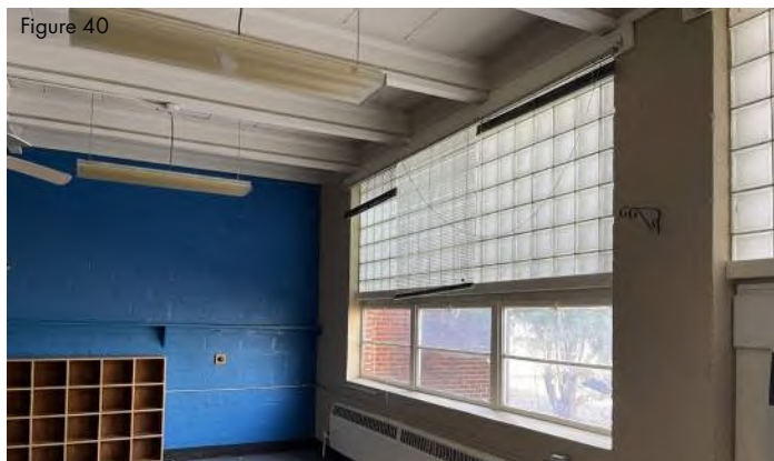
Typical exposed ceiling in classrooms - underside of concrete roof deck & concrete joists
