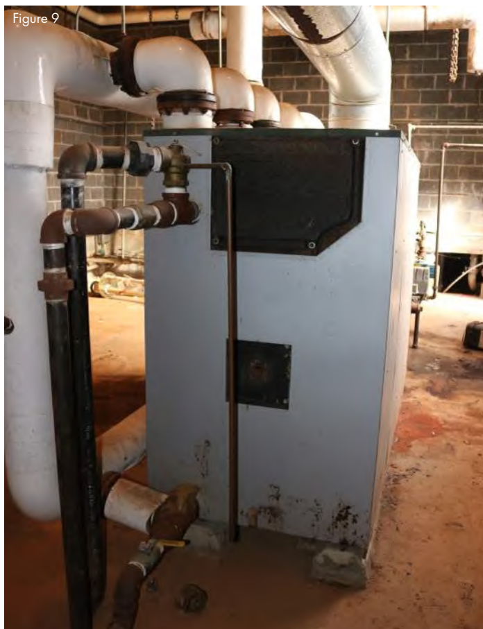
Back side of boiler. Cabinet is rusting.
