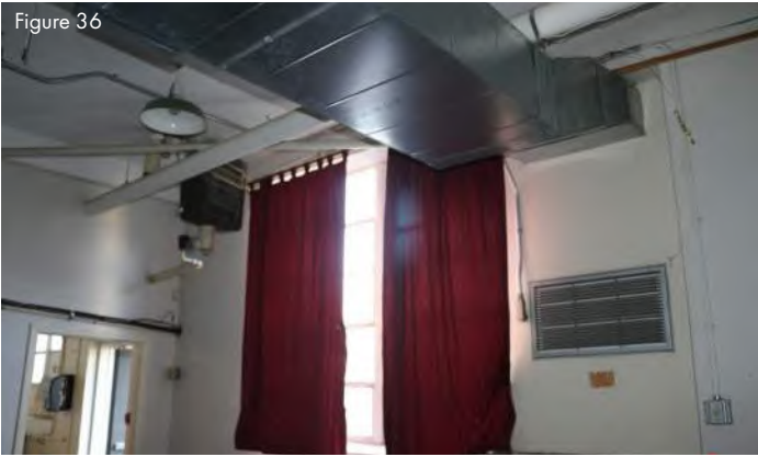
Lower-level Gym office area served by Bard unit. Steam unit heater in the background.
