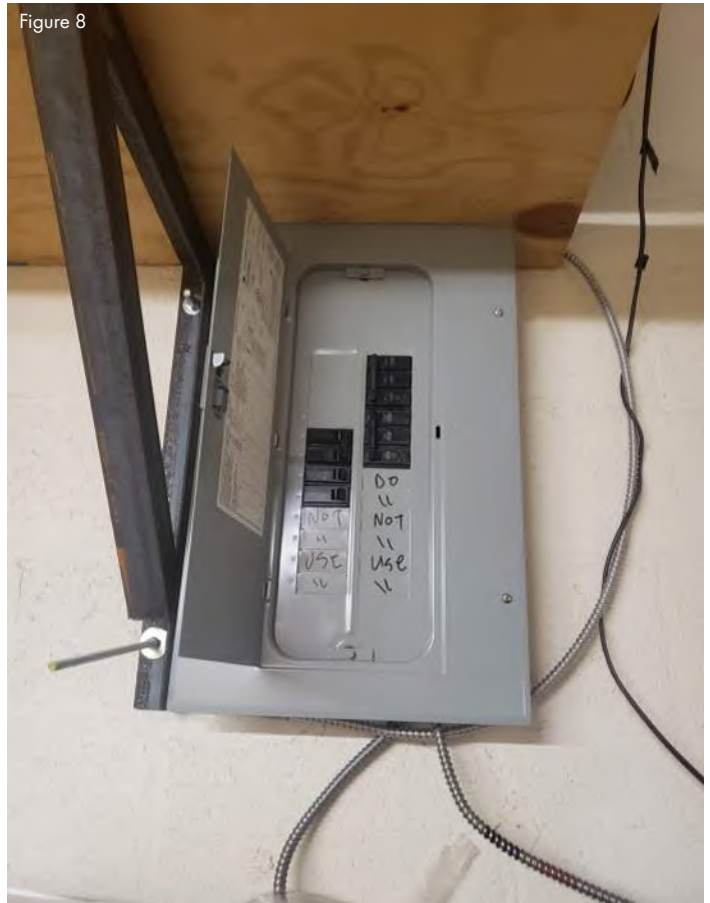
Electrical panel located directly under an air handling unit.
