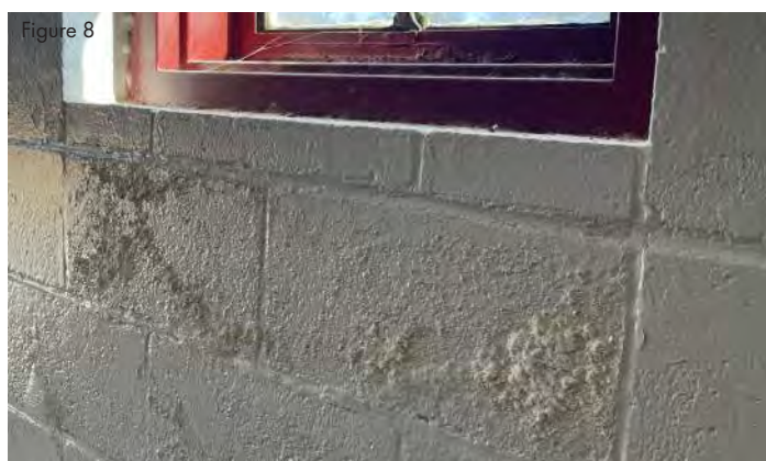
Evidence of moisture infiltration in addition stairwell
