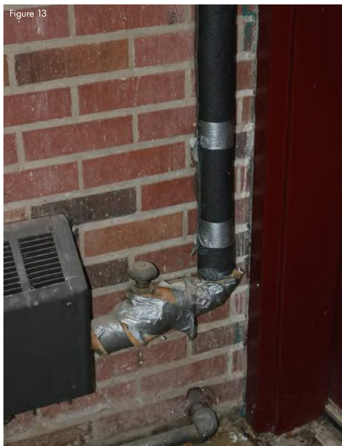
The radiator at bottom of classroom stairwell needs to have pipe insulation replaced.
