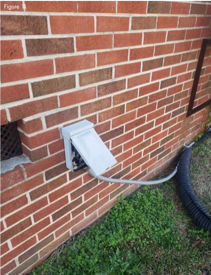
Exterior disconnect is missing interior escutcheon to conceal the wiring and is open to the elements.
