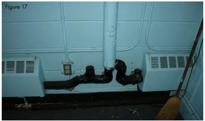
Lower-level classroom stairwell needs to have pipe insulation replaced.
