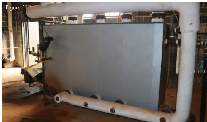
Hot water/Steam pipe insulation in various conditions. Some sections need to be replaced.
