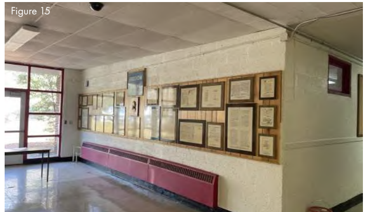
ACP ceiling in fair condition - notice bending of the panel edges
